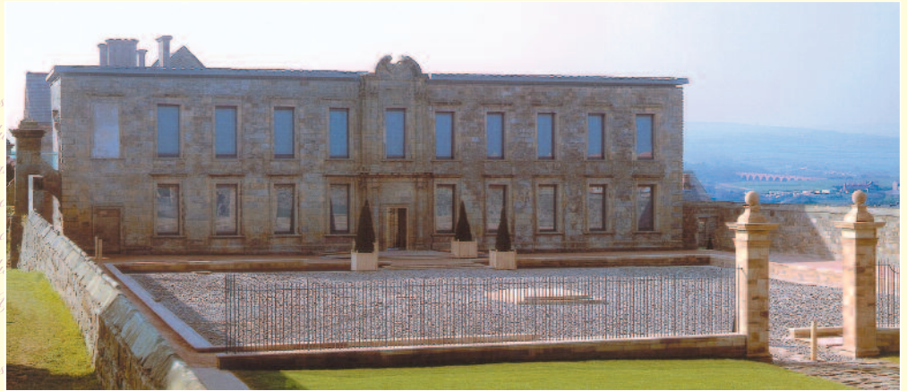
Whitby Abbey Banqueting Hall. Conversion to visitor centre for English Heritage
