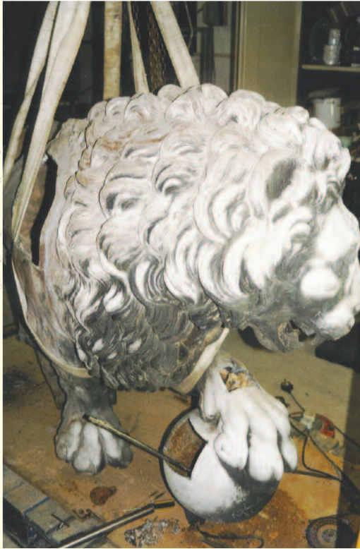
Medici Lion head undergoing internal strengthening to avoid collapse
