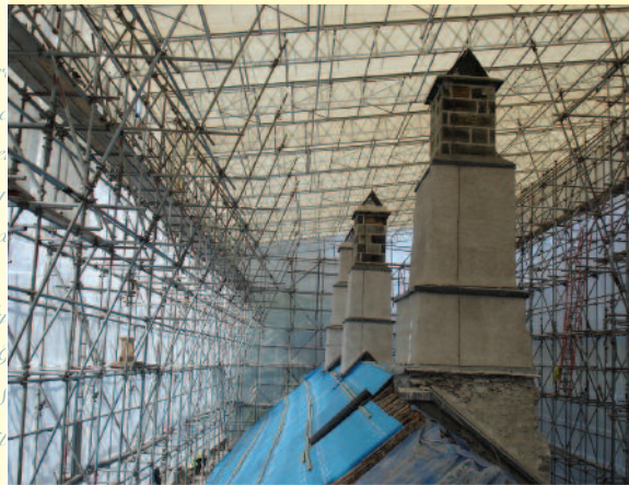
Sizergh Castle roof repairs
