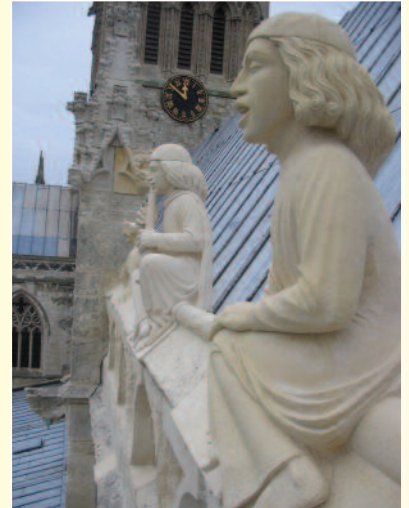
Selby Abbey Stonework conservation and repair
