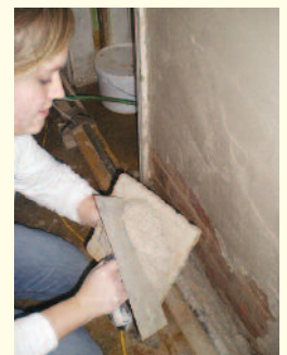
Hands on practical works
